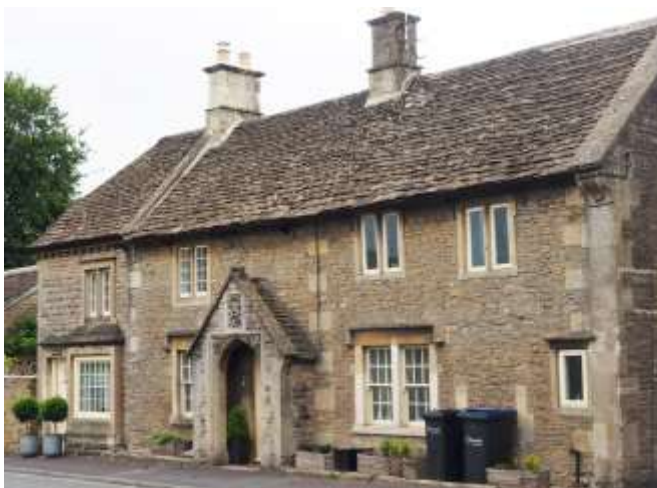
Poynder porch added to older house
