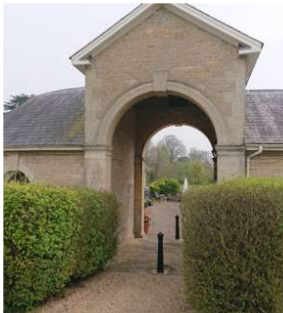
The arch through the Stables at Beechfield
