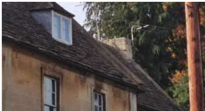
Chimney stump—at far end
