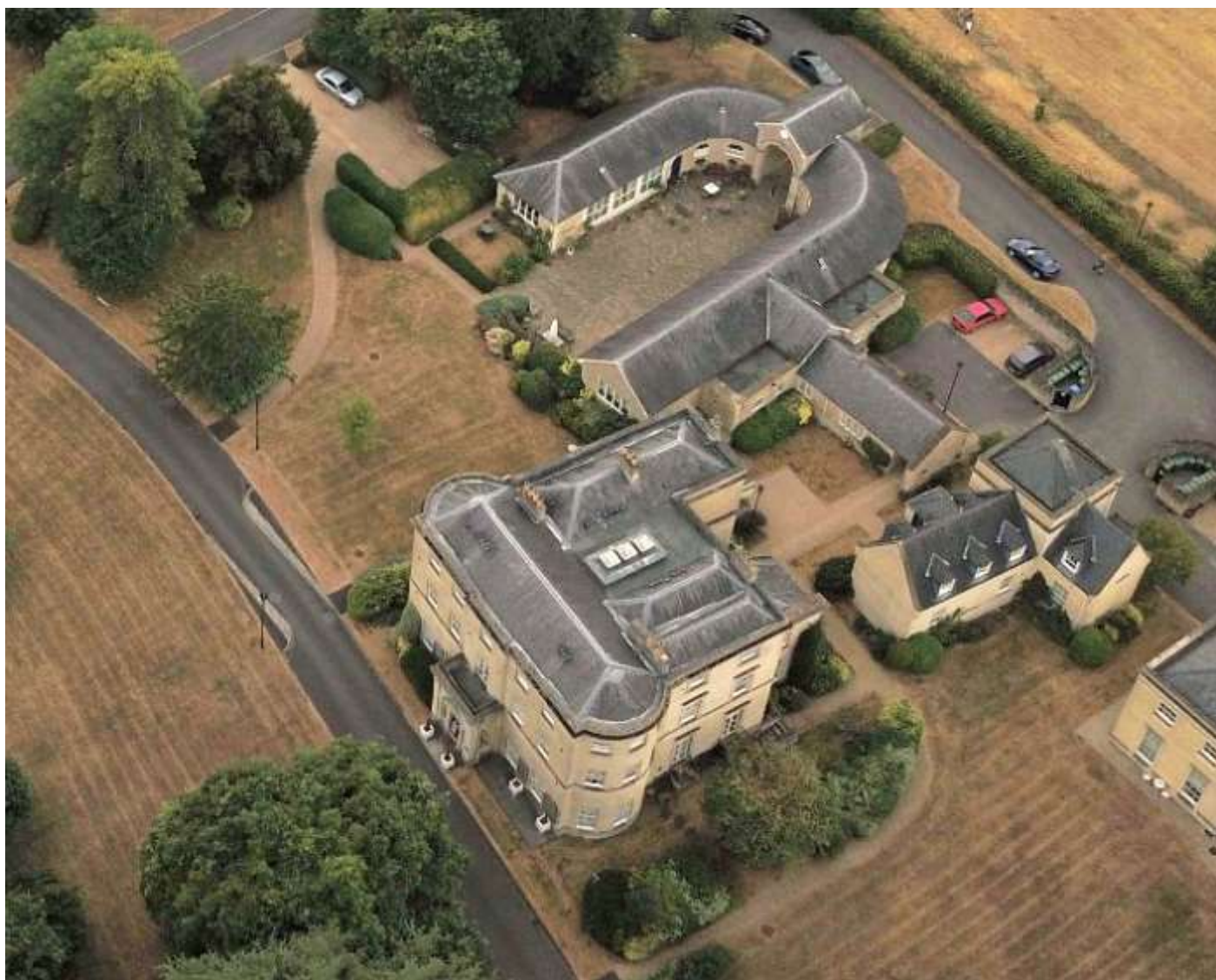
Beechfield House and The Stables
