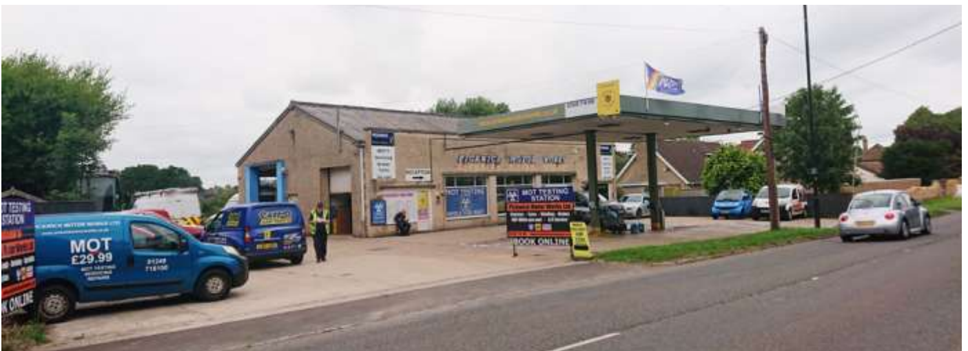
Pickwick Motor Works
